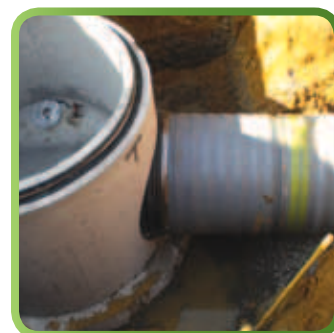
Boot Connection Directly to SaniTite HP
