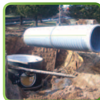
A-Lok Premium Compression Connection
